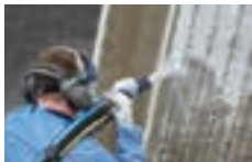
8.6 to 10 bar: Abrasive blasting
